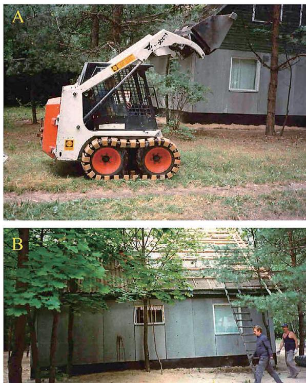
Fig. 6 “Bobcat” minibulldozer is ready to start top-soil removal around house No. 1 in Muravinka (A). Roof replacement on house No. 1 in Muravinka after top-soil removal and application of clean sand (B).
