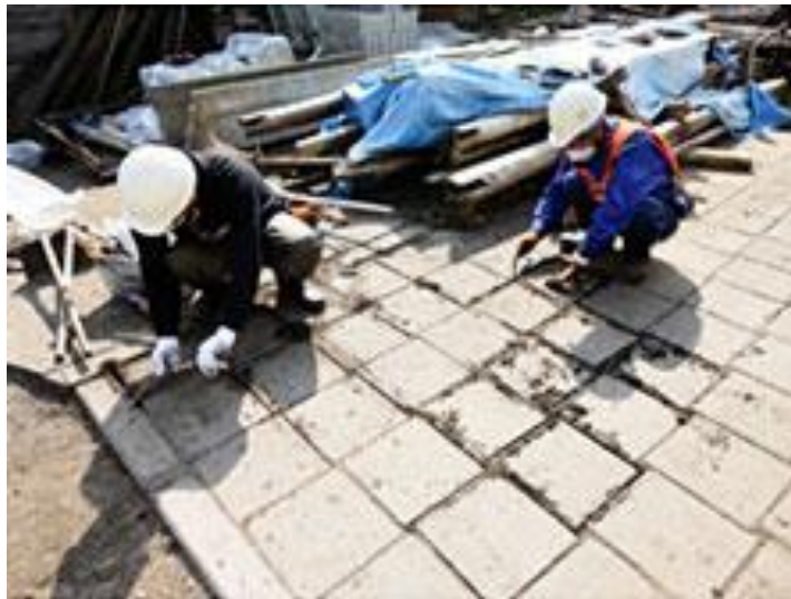
ground : Removal of deposited materials
